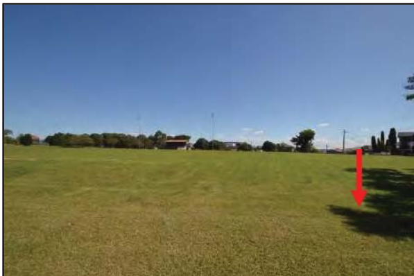
Figure 8. The oval as seen from the east, approximate location of proposed lighting poles indicated by arrow.
